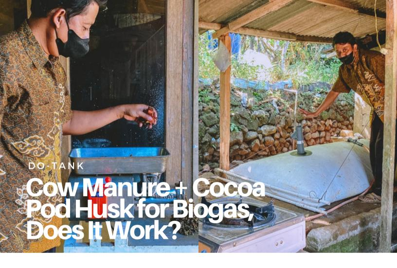
After installing a biogas digester at Pak Paryanto's place in Gunung Kidul, Yogyakarta, we keep maintaining the progress of this biogas. This biogas is unique as usually, our biogas is fed with only cow manure. su-re.co, in collaboration with Universitas Gadjah Mada, analyzed the efficacy of cacao pod husk (CPH) and cow manure to feed the biogas. We conducted this analysis to turn waste into energy using the agricultural waste produced by Pak Paryanto's cacao farm.
