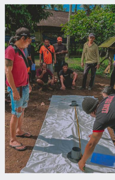
Kadek Kudana is one of the cacao farmers who received a biogas digester. He even installed the biogas himself! Unlike the usual feedstock, Pak Kadek feeds his biogas with pig manure; surprisingly, it works very well! His biogas stove has produced a big blue fire that can last up to one hour daily. Other than that, Pak Kadek and the other farmers also have some bio-slurry that works as organic fertiliser.
