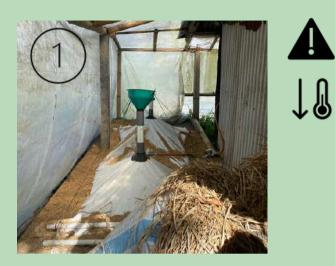
Biogas digesters produce less gas in **cooler environments**.
